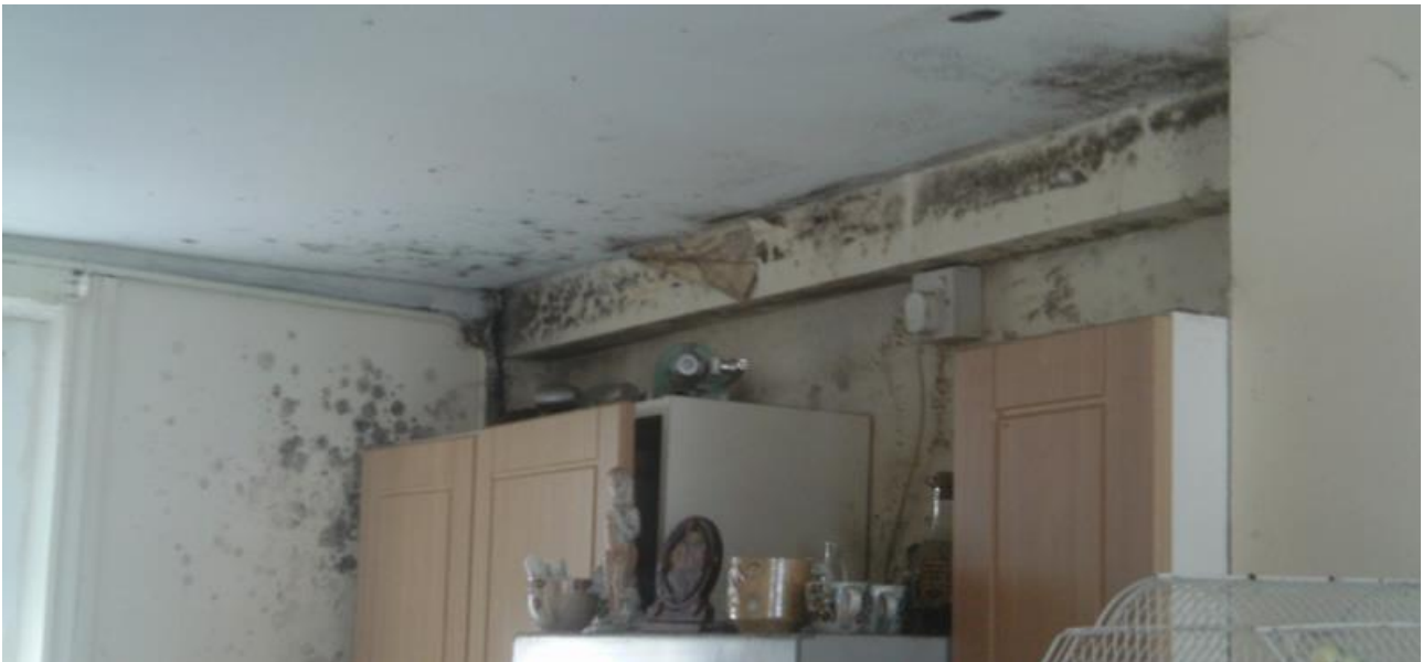
Figure 1: This kitchen of a mid-terrace home in Crecora Avenue, Ballinacurra Weston, which was newly installed and decorated in 2011, shows the effect caused by penetrating damp from the adjoining boarded-up house in 2013
